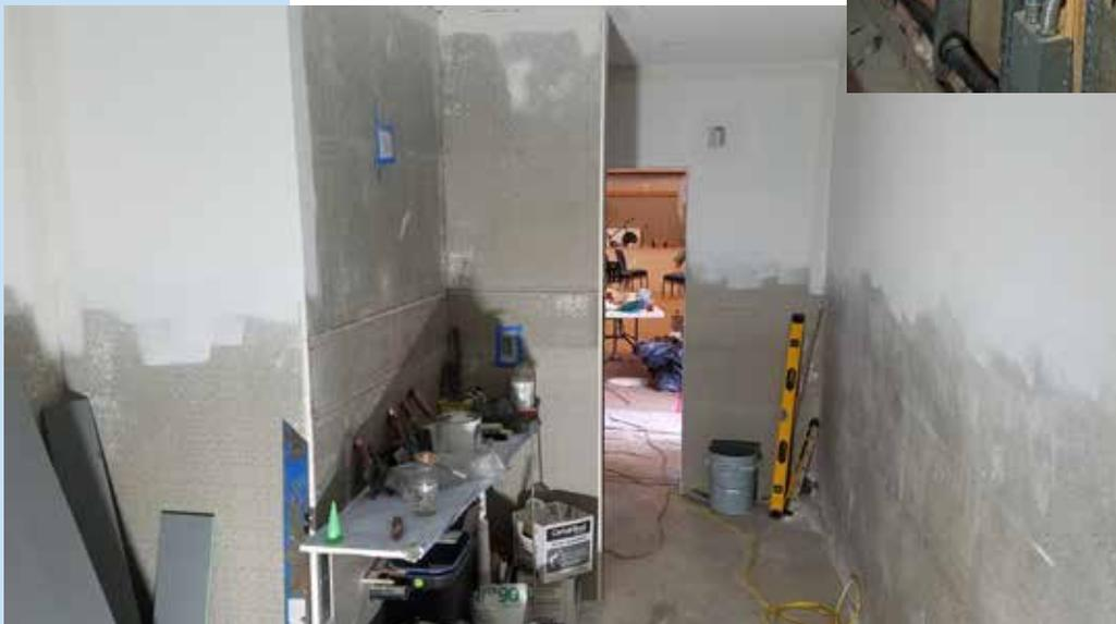
(at left) Preparation underway for wall tile. All 3 bathrooms will have 4x8-foot wall tile from floor to about door height, with a contrasting vertical stripe of mixed tile for interest.
